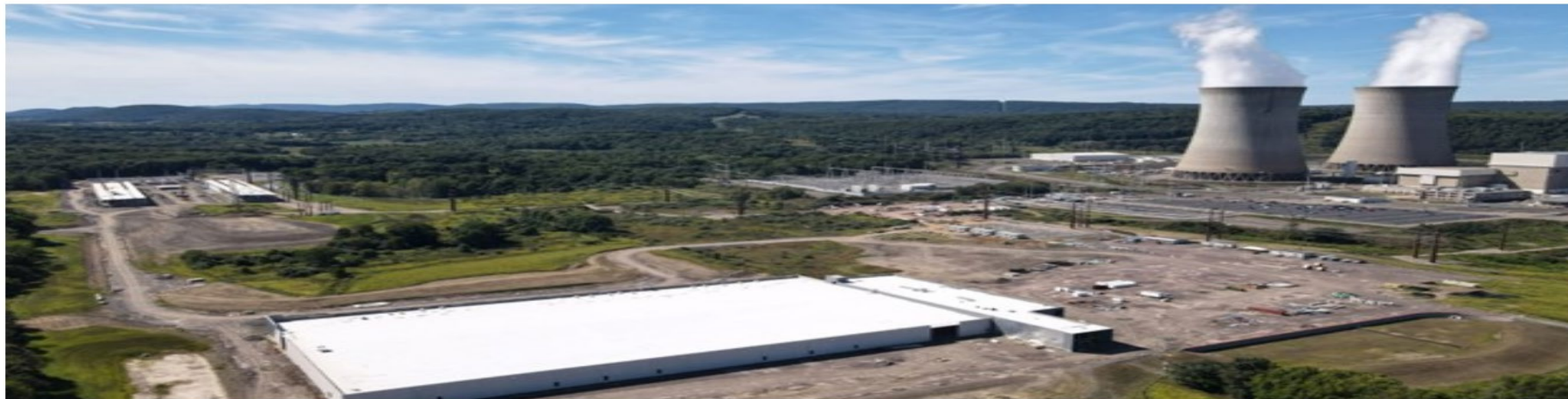
Susquehanna nuclear plant in Salem Township, Penn., along with the data center in foreground. (Photo: Talen Energy)
